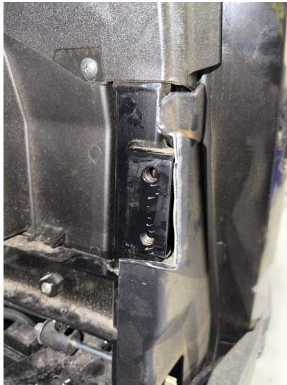
FIG 3 - Lower Cab mount exposed after trimming
