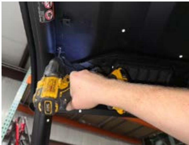
FIG 11 - Drill Front Mount Holes
