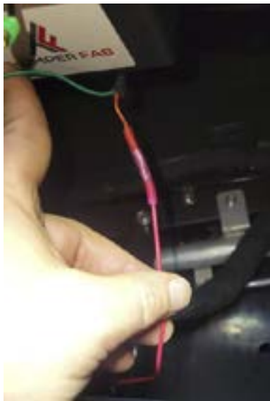
FIG 16 - Splice wires together
