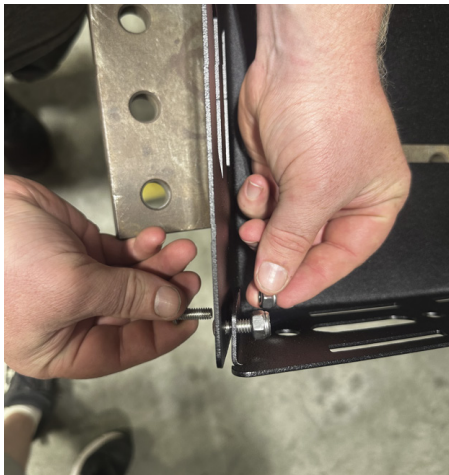
FIG 9 - Fasten flanges of Top Basket together
