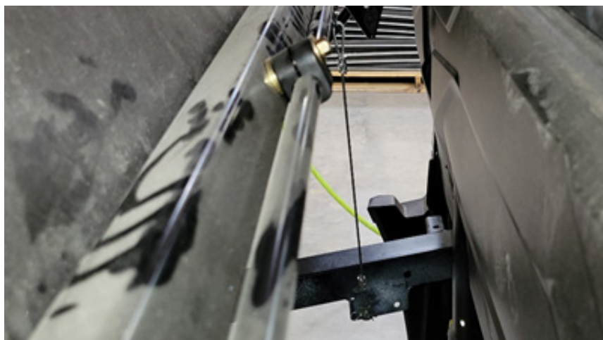
FIG 12 - Install Retention Cable Frame Mount
