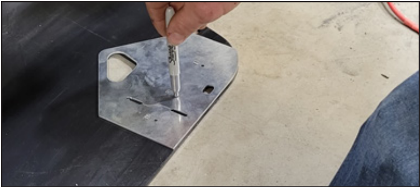
FIG 2 - Use Template to mark front hole using “F” hole on template.
