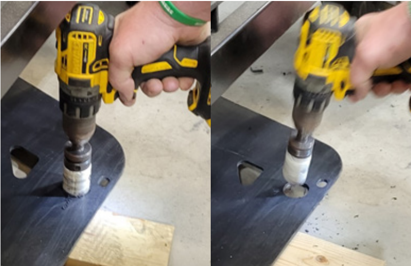
FIG 5 - Cut holes out of skidplate using 1.5" Holesaw.
