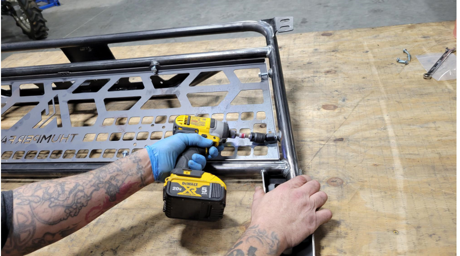
FIG 1 - Fasten Accent Panel To Headache Rack Using 13 mm Socket
