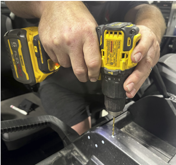
FIG 2 - Drill pilot holes with 1/8" Drill Bit
