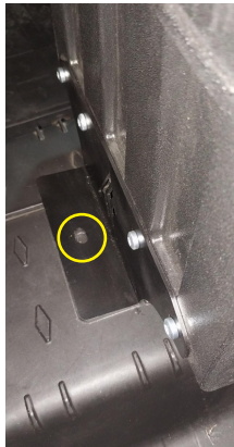
FIG 9 - Fasten L-Bracket to the floor using a drill
