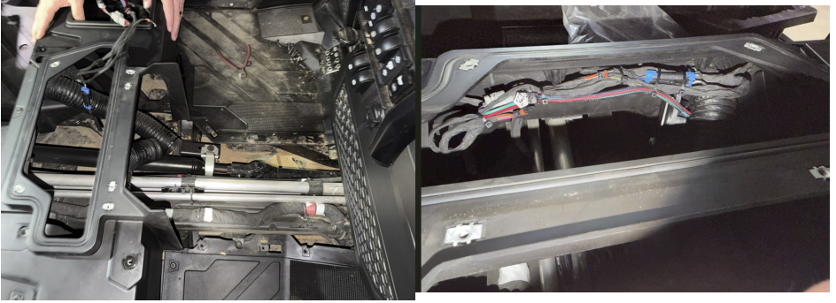
FIG 32 & FIG 33 - Route harness to inside seat cubby and zip tie wires together
